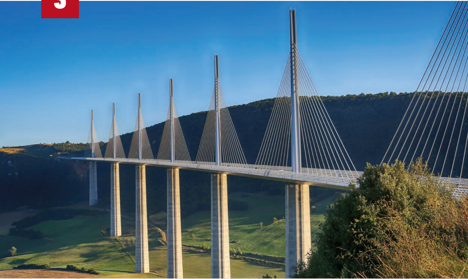
Millau Viaduct, Aveyron, France
